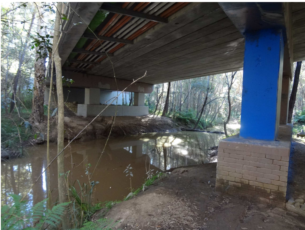
Blunder Creek – upstream side of the bridge (left hand side)
