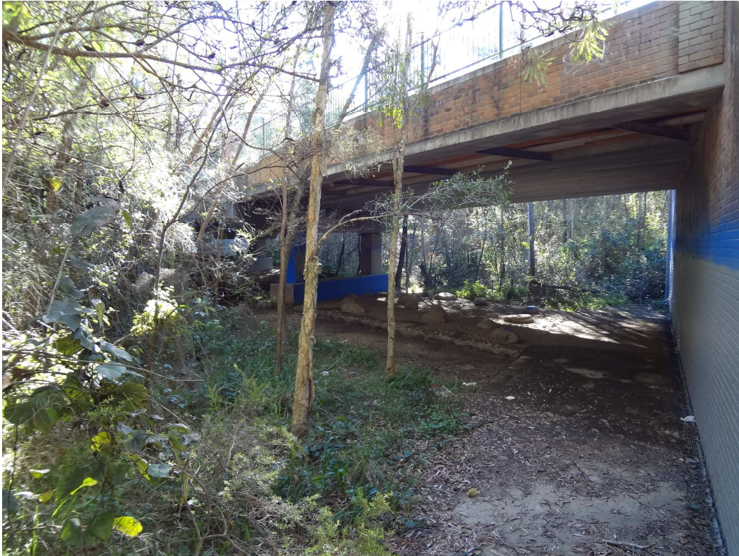
Blunder Creek – upstream side of the bridge (right hand side)
