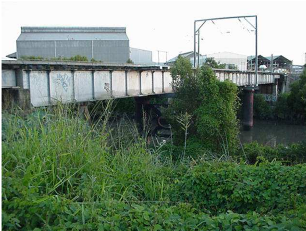
Oxley Creek – Downstream Looking Upstream at Railway Crossing
