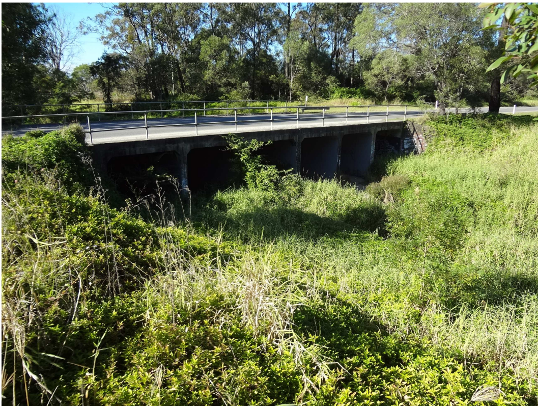
Sheepstation Creek – downstream side of the culvert
