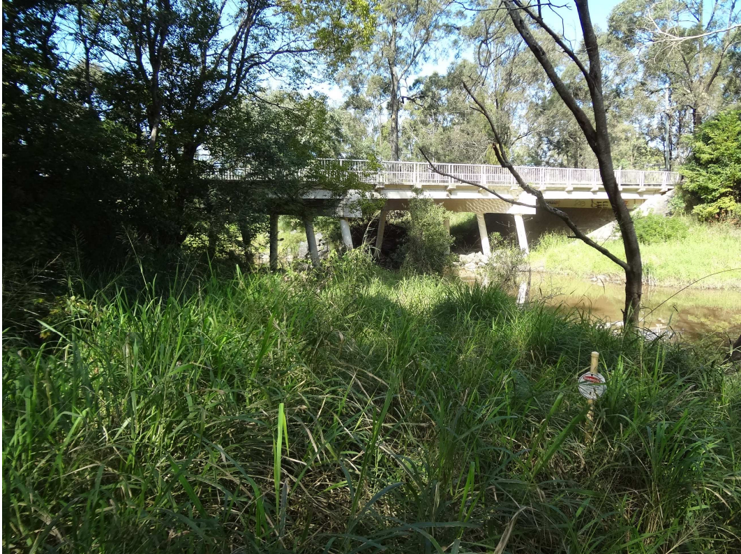
Oxley Creek – downstream side of the bridge
