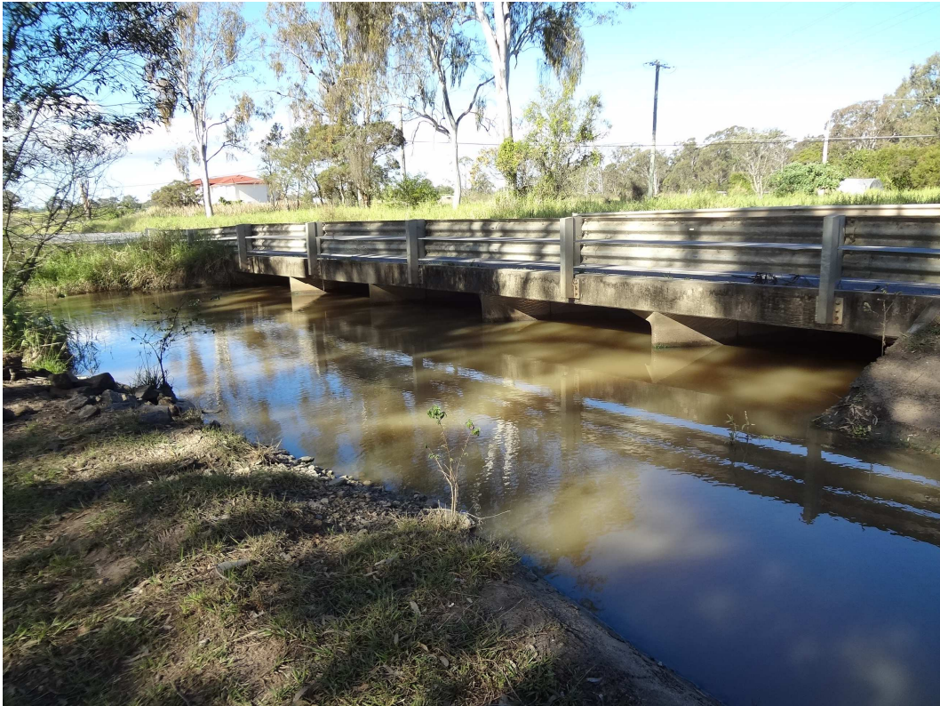
Blunder Creek – downstream side of the culvert
