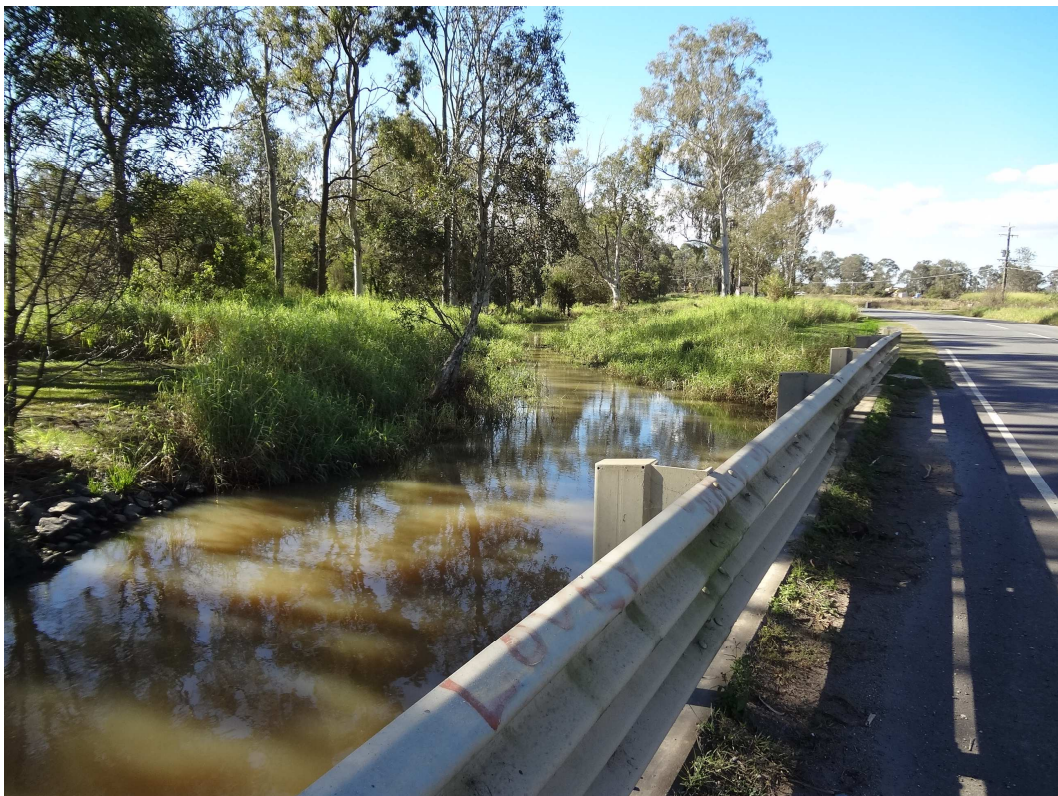
Blunder Creek – stand on the culvert looking downstream
