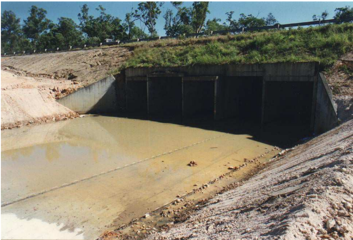
Blunder Creek – upstream side of the culvert
