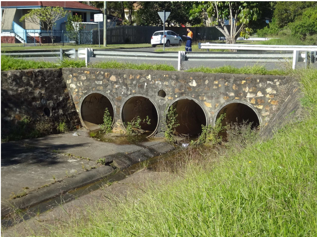
Blunder Creek Tributary – downstream side of the culvert
