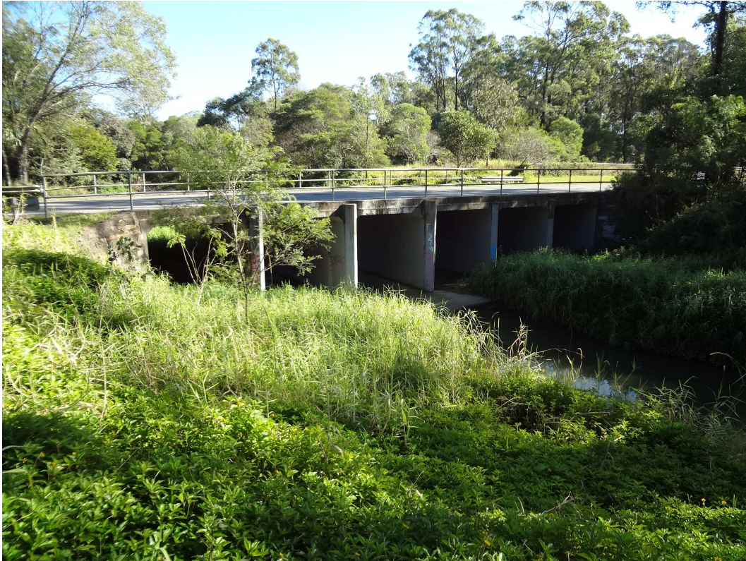
Sheepstation Creek – upstream side of the culvert
