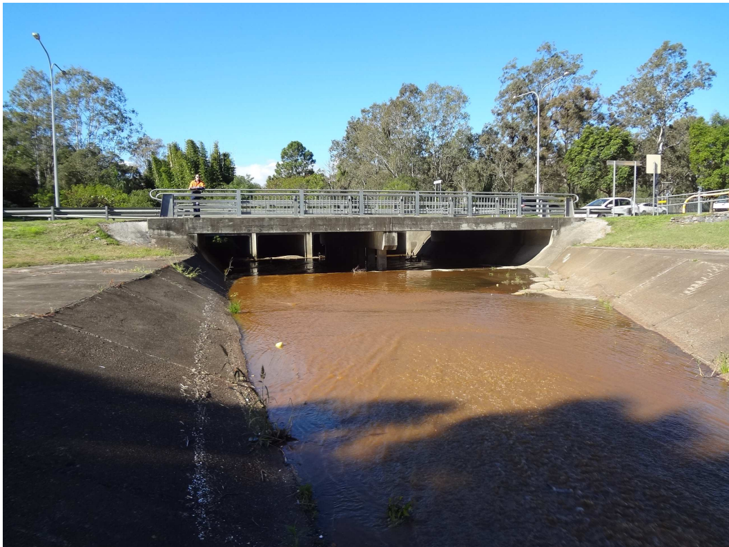
Blunder Creek Tributary – upstream side of the bridge
