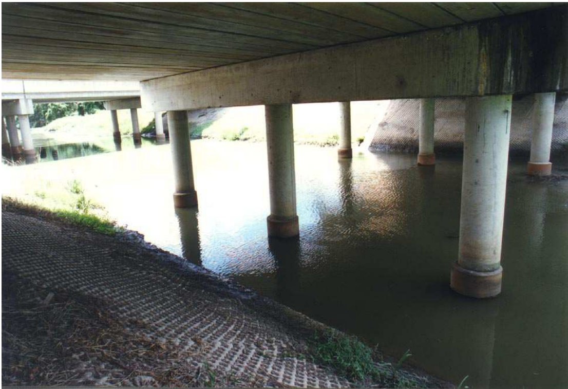
Oxley Creek – Under Ipswich Road Looking Downstream
