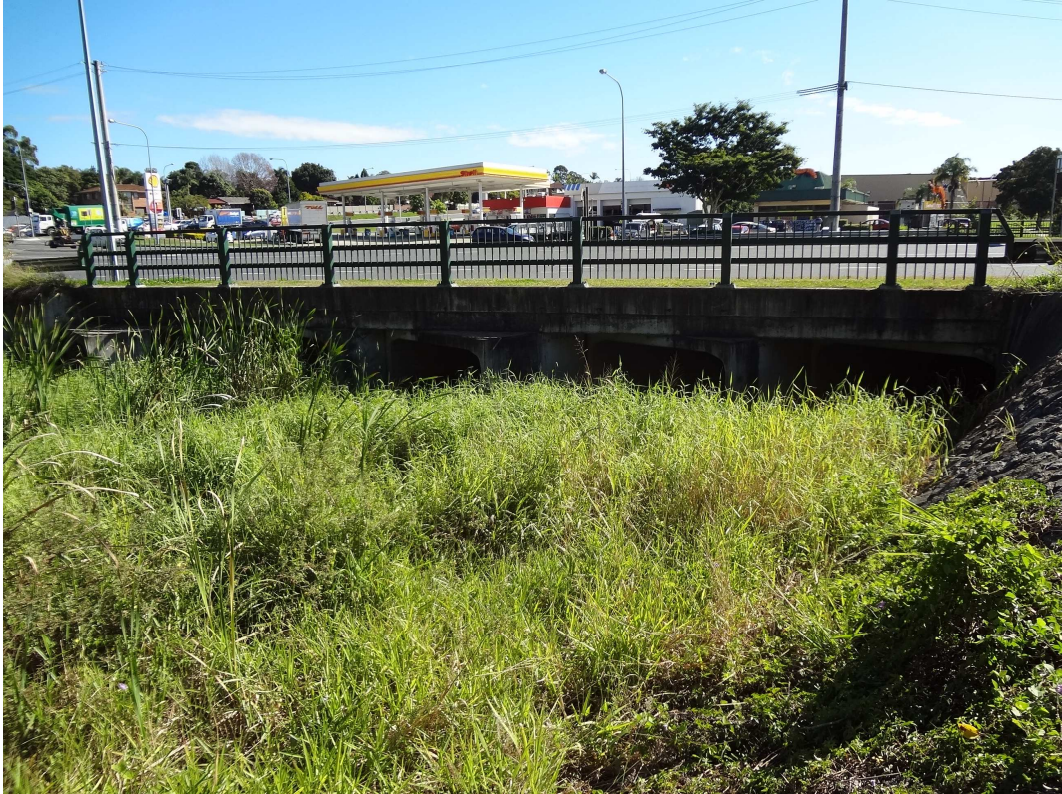
Blunder Creek Tributary – upstream side of the culvert
