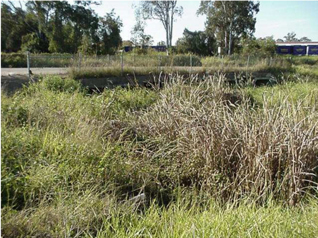
Oxley Creek Tributary – upstream side of the culvert
