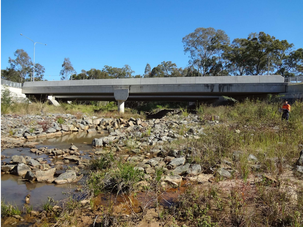
Blunder Creek – downstream side of the bridge
