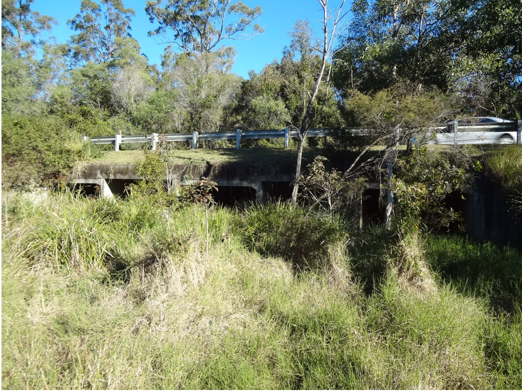
Blunder Creek – downstream side of the culvert
