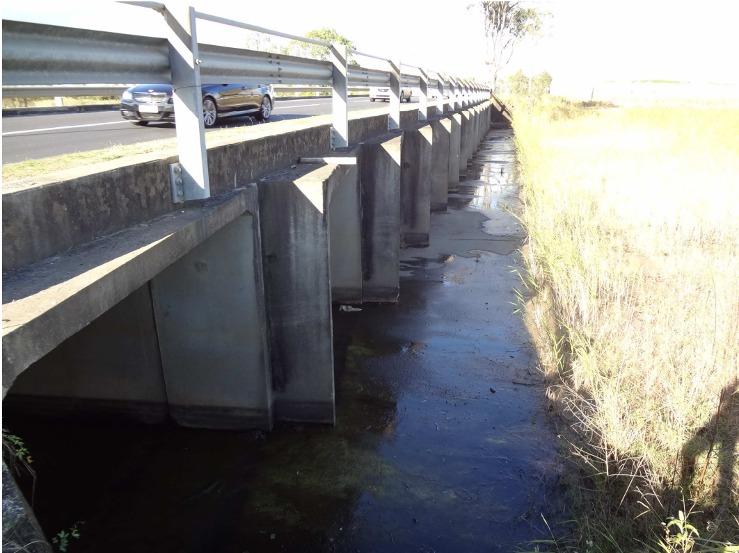
Oxley Creek – upstream side of the culvert
