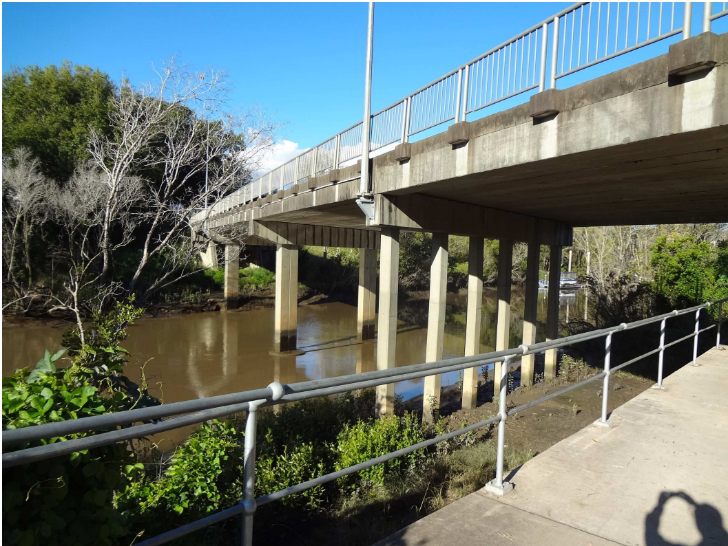
Oxley Creek – downstream side of the bridge
