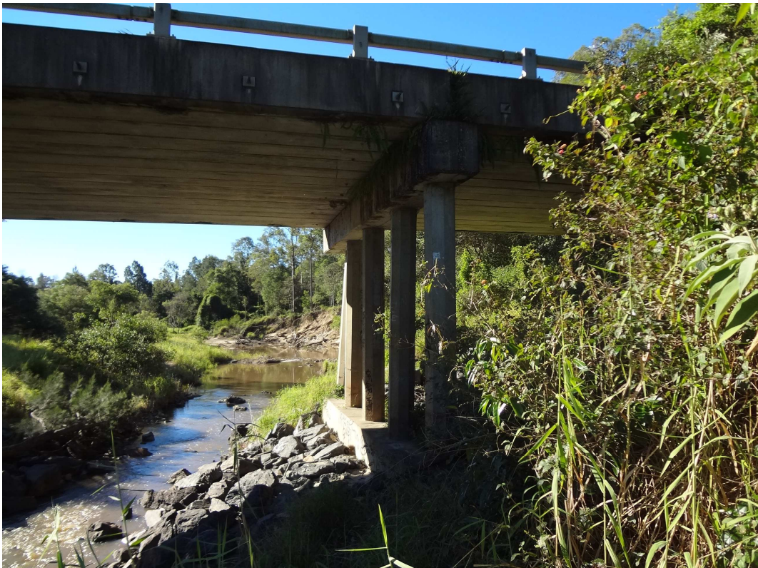
Oxley Creek – upstream side of the bridge (right hand side)
