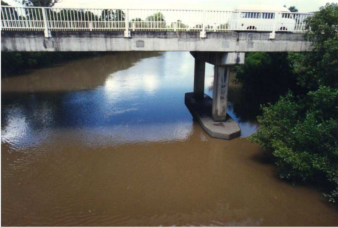
Oxley Creek – Downstream Looking Upstream at Sherwood Road
