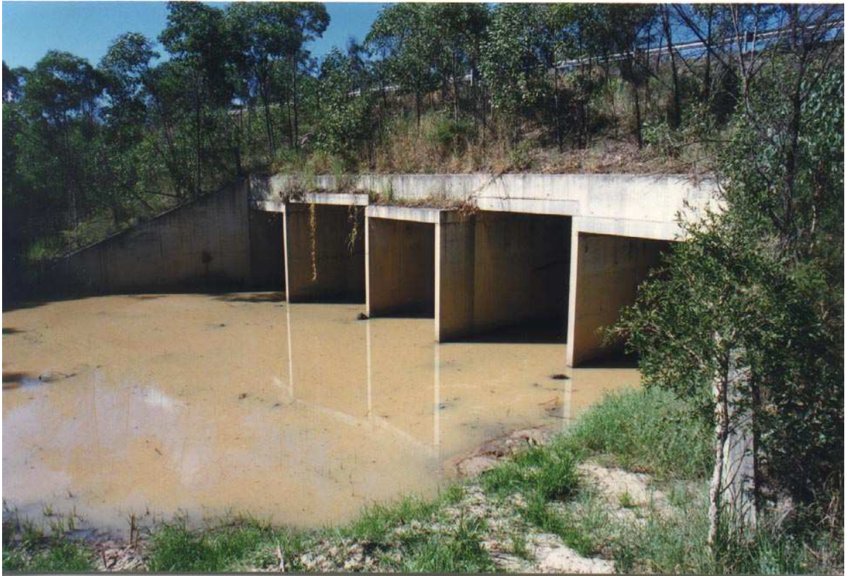
Blunder Creek – downstream side of the culvert
