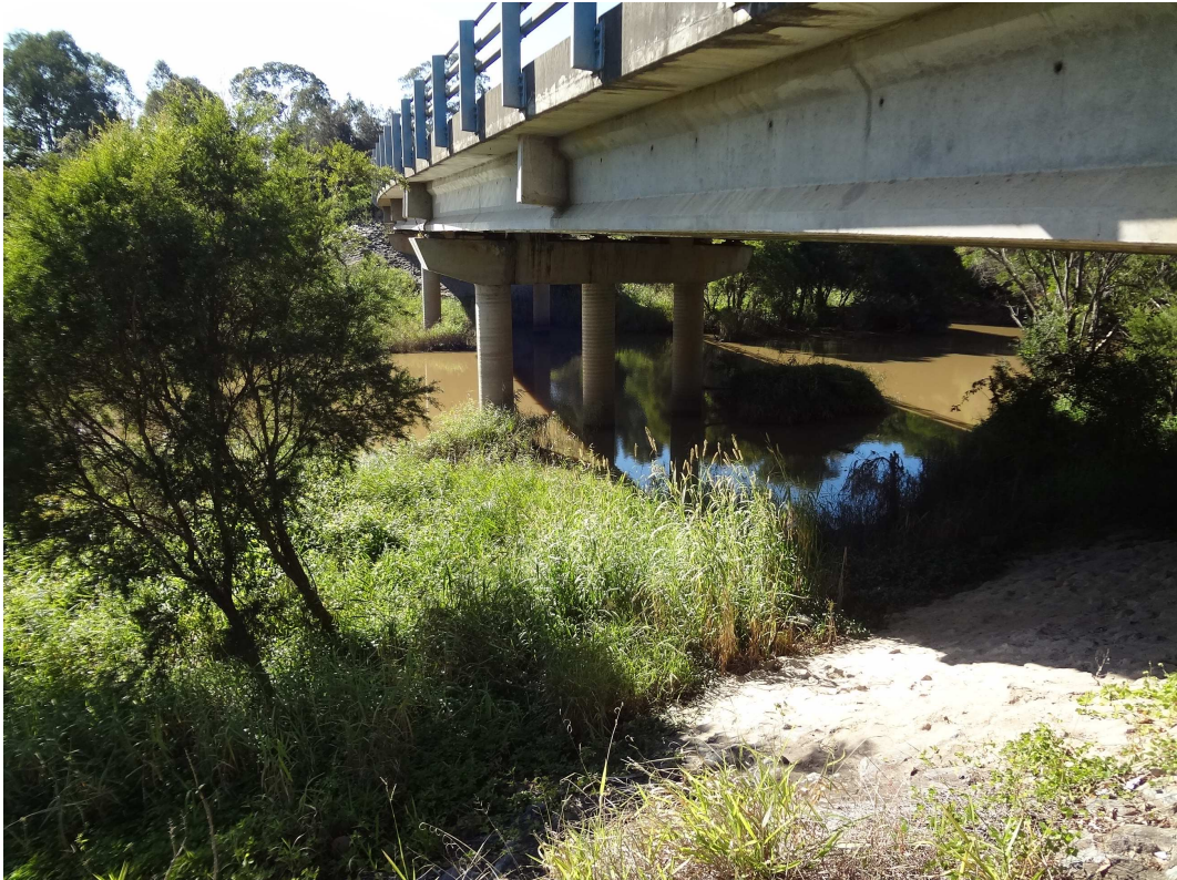
Oxley Creek – downstream side of the bridge
