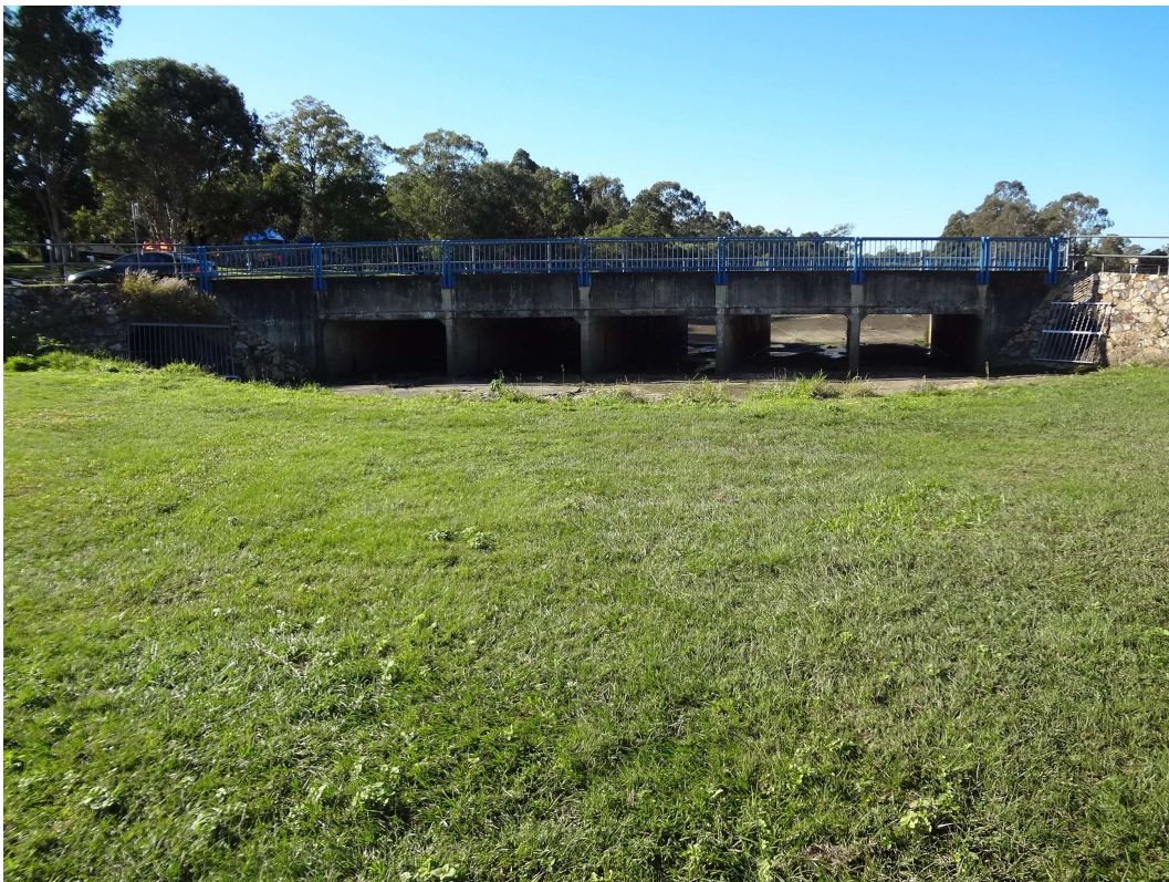
Sheepstation Creek – downstream side of the culvert
