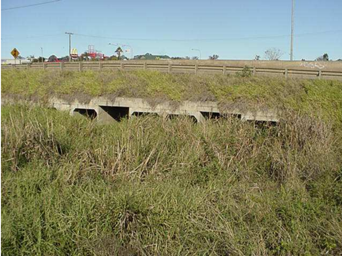
Oxley Creek Tributary – downstream side of the culvert
