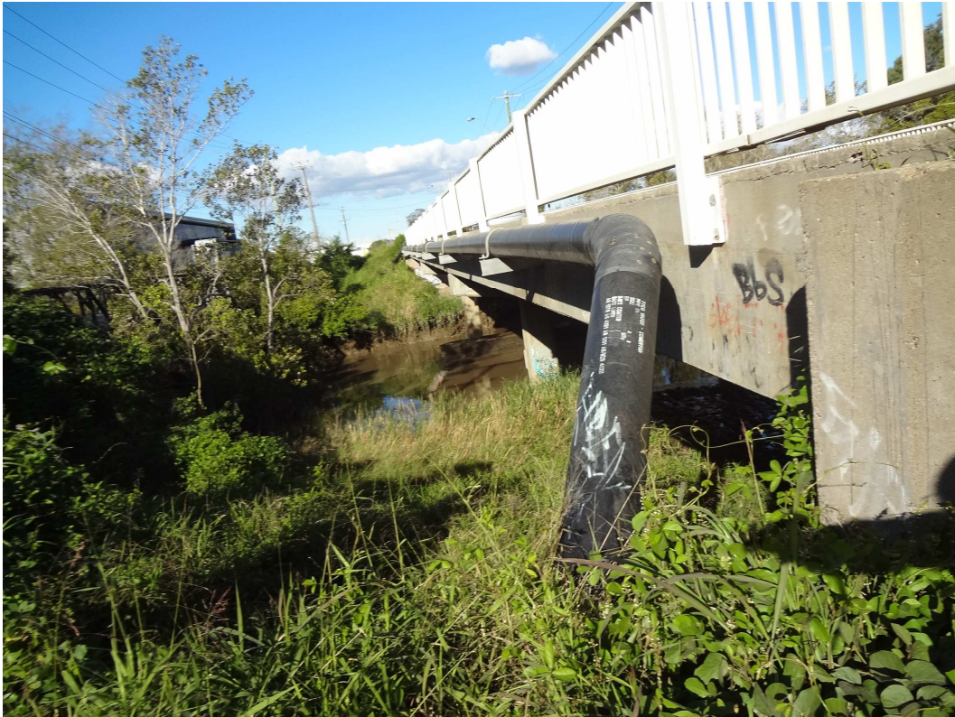
Oxley Creek – downstream side of the bridge
