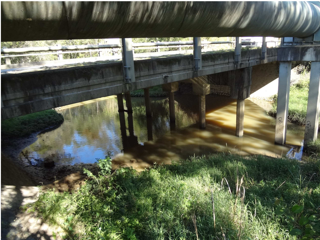
Blunder Creek – downstream side of the bridge
