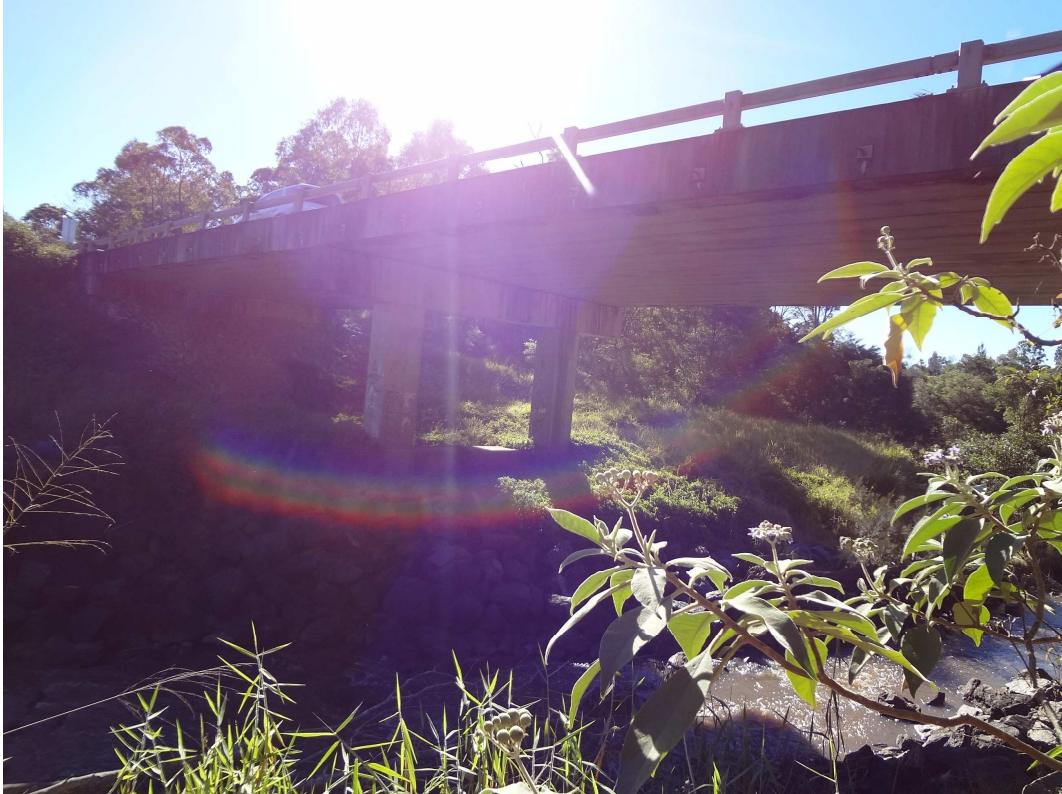
Oxley Creek – upstream side of the bridge (left hand side)
