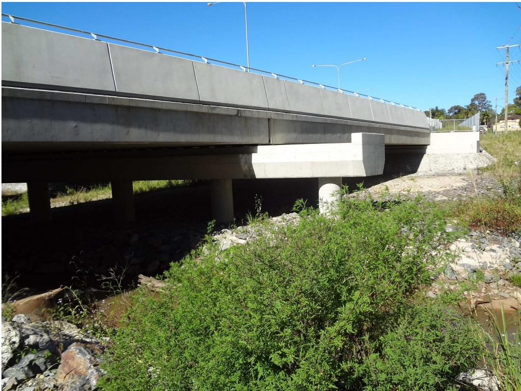
Blunder Creek – upstream side of the bridge
