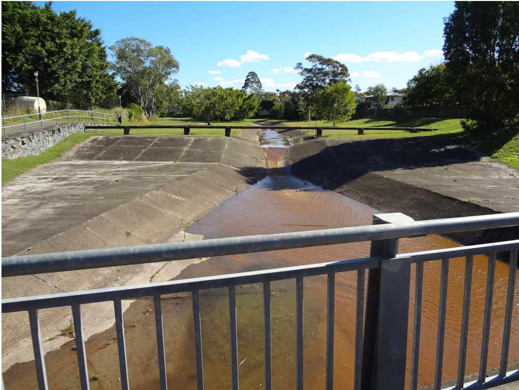
Blunder Creek Tributary – stand on the bridge looking upstream
