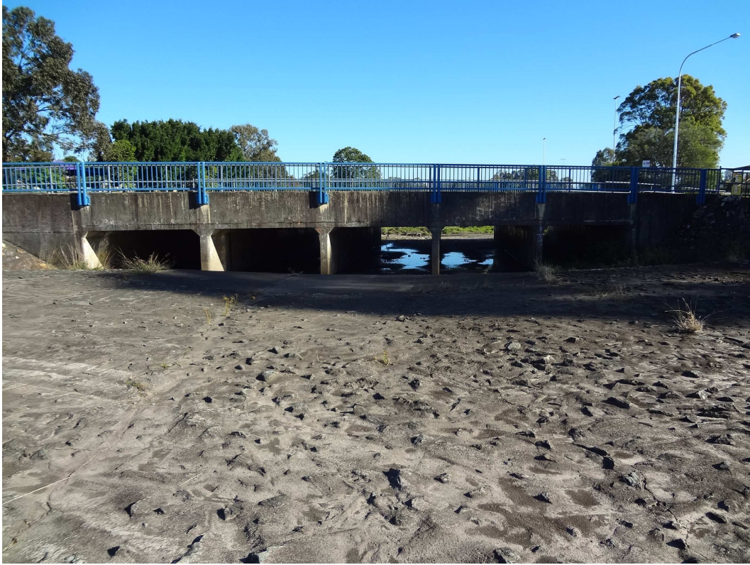
Sheepstation Creek – upstream side of the culvert
